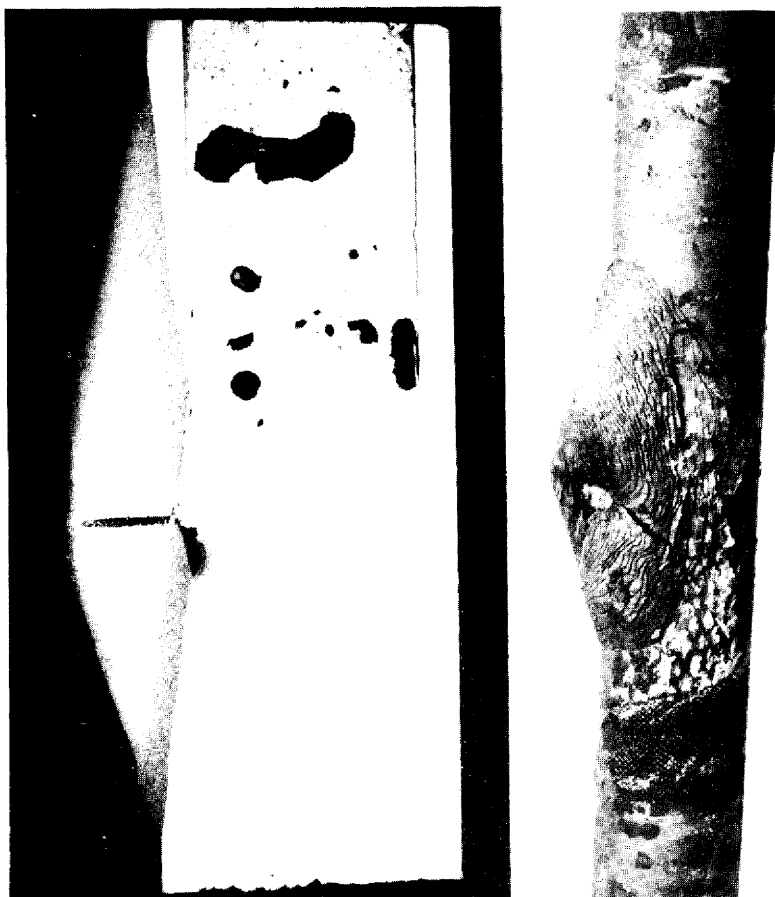
FIG. 21-11. Rapid oxidation of 2 \frac{1}{4} % G-1% Mo steel pipe after 1025 hr at 594°C at pinhole leak.
