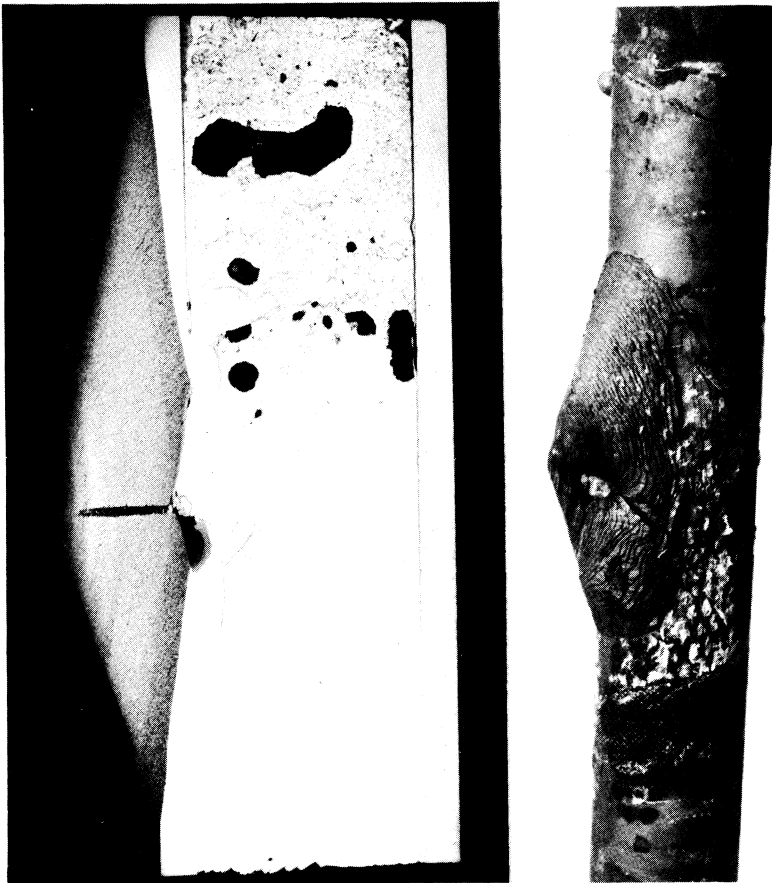
FIG. 21-11. Rapid oxidation of 2¼% G-1% Mo steel pipe after 1025 hr at 594°C at pinhole leak.
