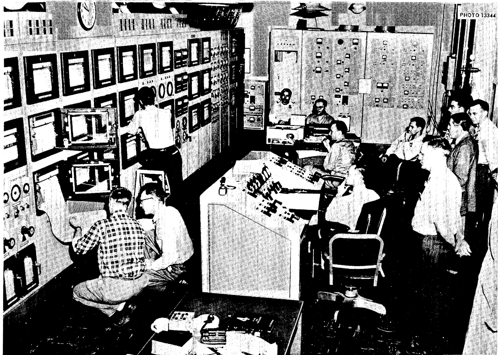
Fig. 5.2. Typical Control Room Scene: Examining Charts During Rod Calibration Experiments.
