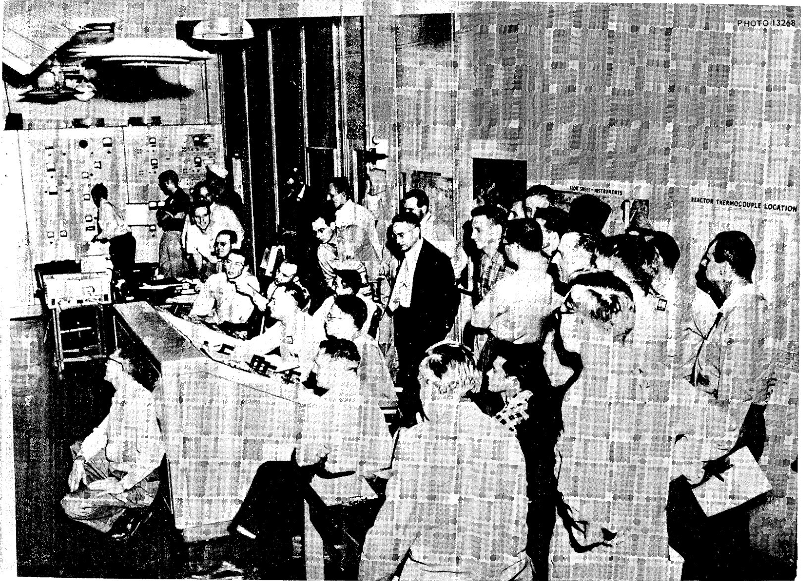
Fig. 4.7. Control Room at Criticality.
