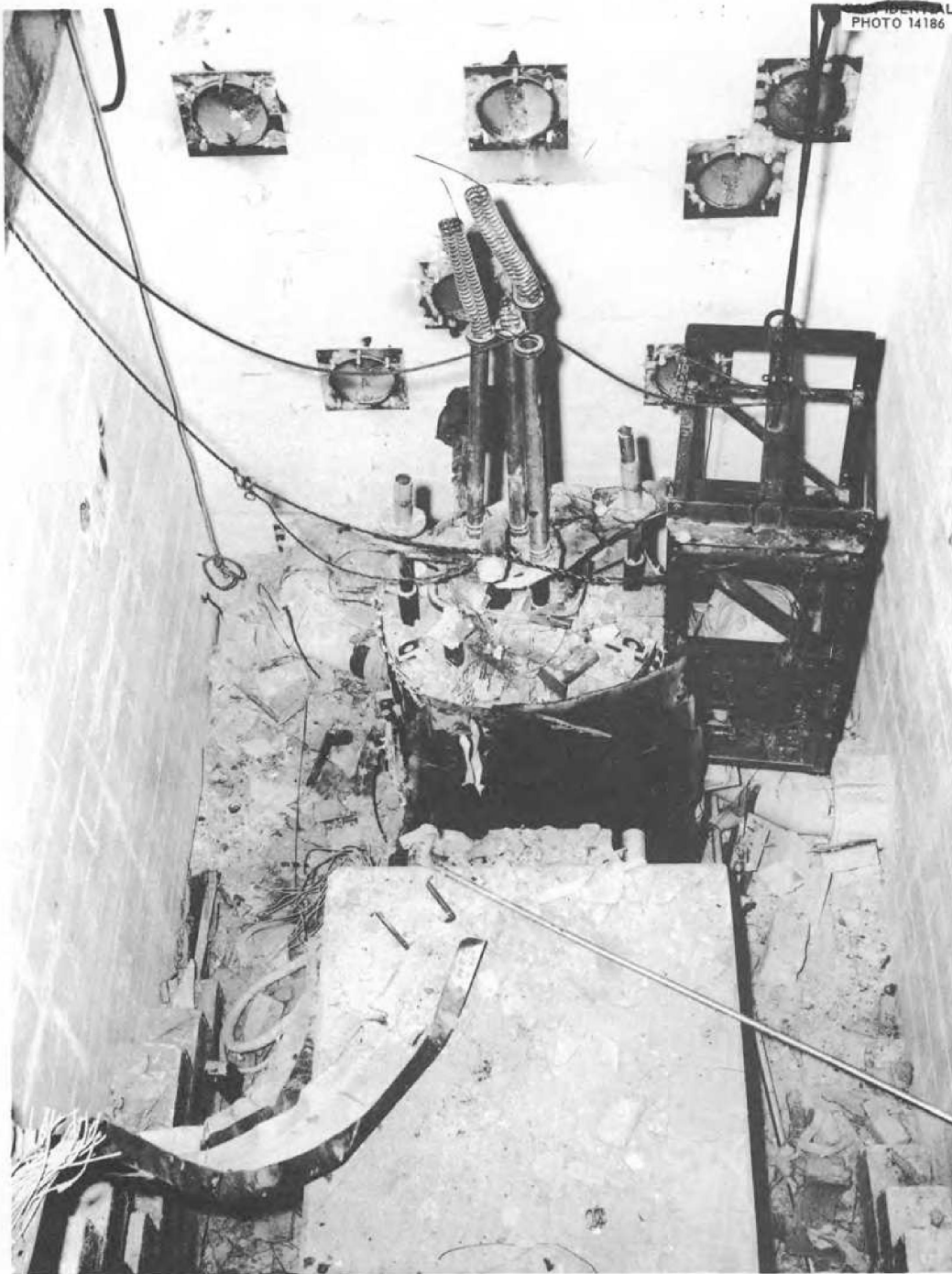
Fig. 9. Gas-Tight Shell Being Removed from Reactor.
