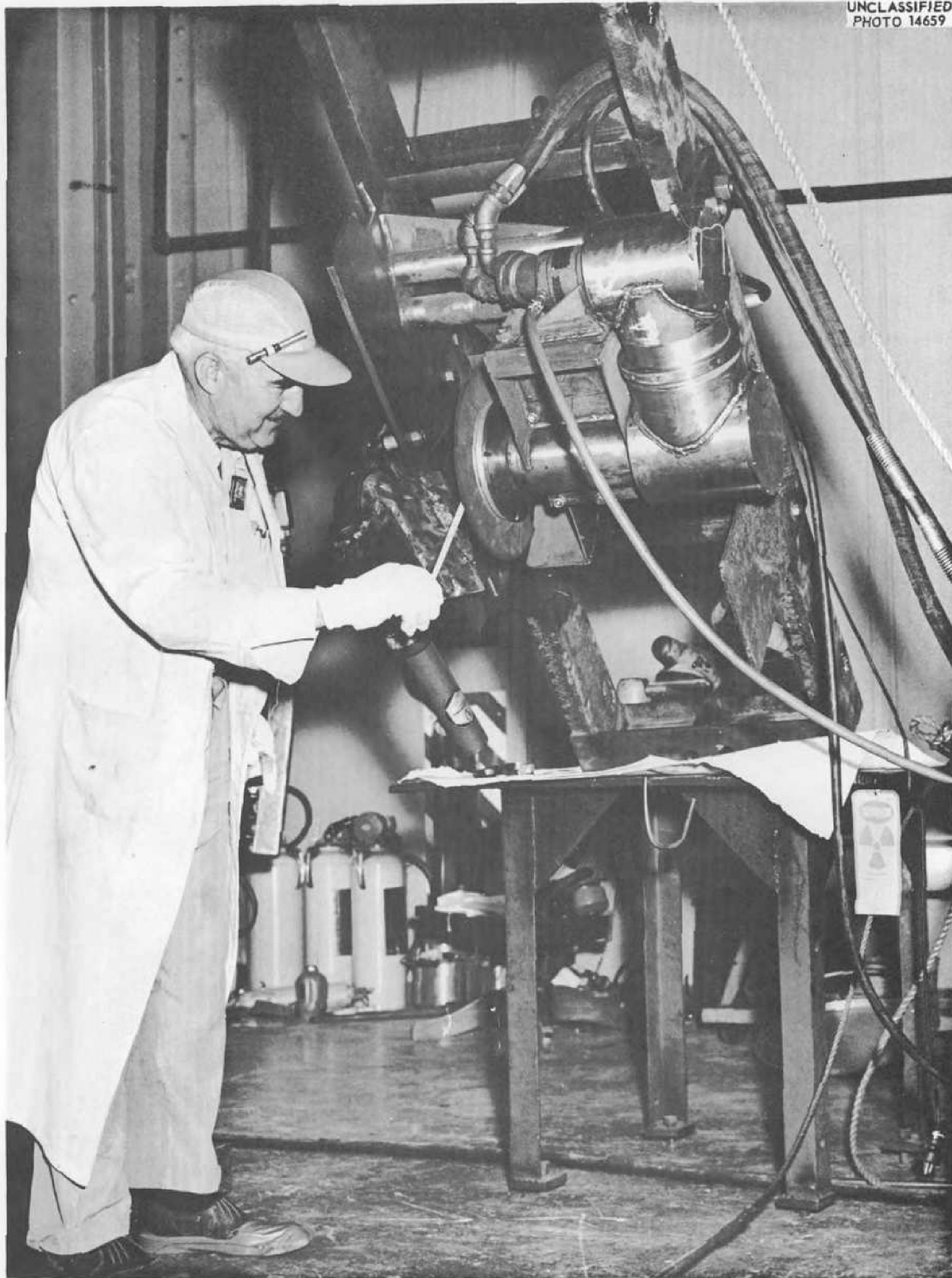
Fig. 11. Cutting Side of Grinder for Dismantling the Reactor.
