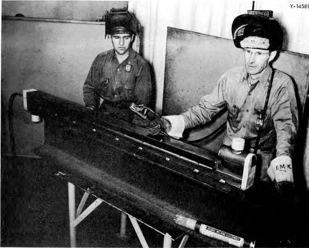
Fig. 15. One Tube Bundle after Completion of Root Weld Pass on Pressure Shell.
