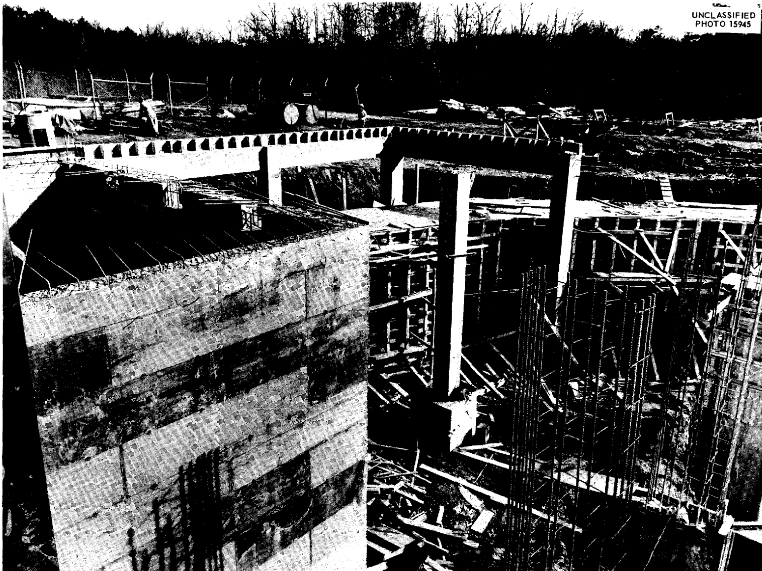
Fig. 1.3. Aircraft Reactor Test Facility Construction as of December 5, 1955, Showing Forms for Spectrometer Tunnel and the Spectrometer Room Wall.
