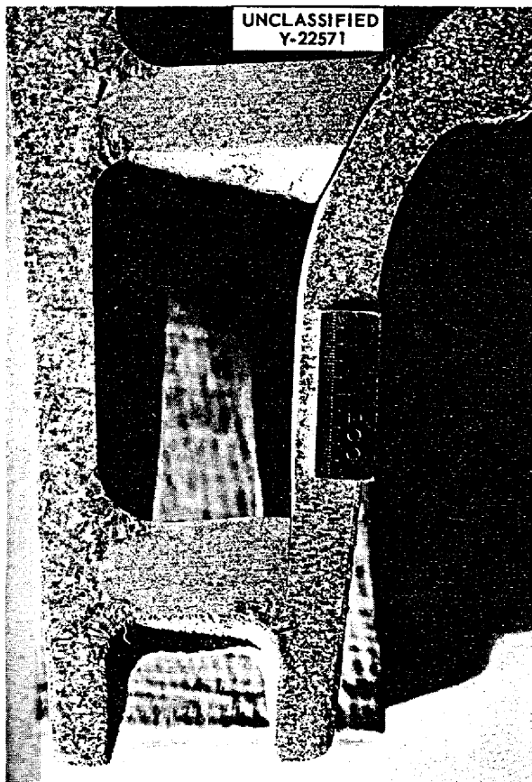
Fig. 3.3.4. Vane-to-Plate Welds of All-Welded Inconel Impeller Fabricated According to Design Shown in Fig. 3.3.3.
