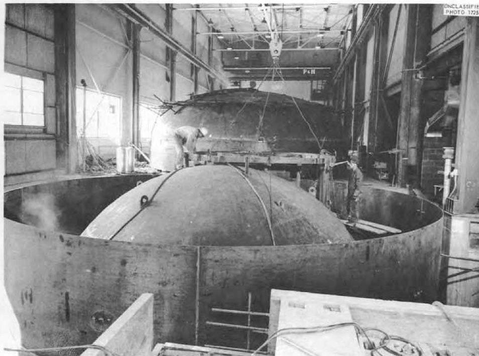
Fig. 1.1.10. Status of Cell Installation in Late March 1956.
