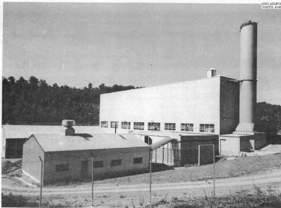
Fig. 20. View of the ART Facility from the Southwest. Photograph showing the present status of the facility. The metal building in the background is the diesel generator house. The compressor house is in the foreground.
