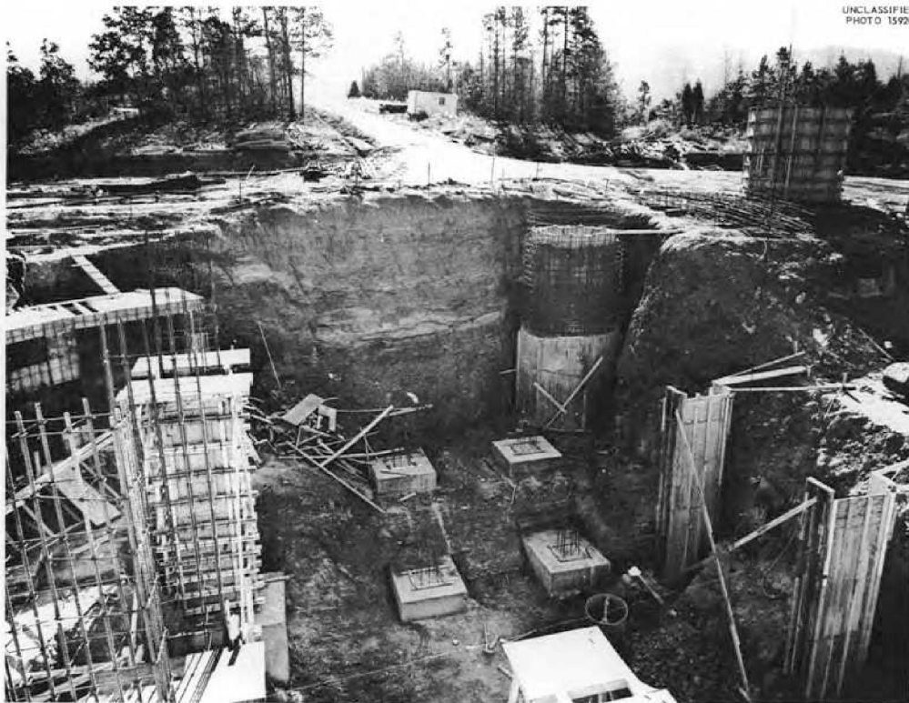
Fig. 6. View from the South End of the Crane Bay of the Original Building 7503. In the right background can be seen the adsorber pit. In the left background can be seen the forms for the walls of the spectrometer tunnel.
