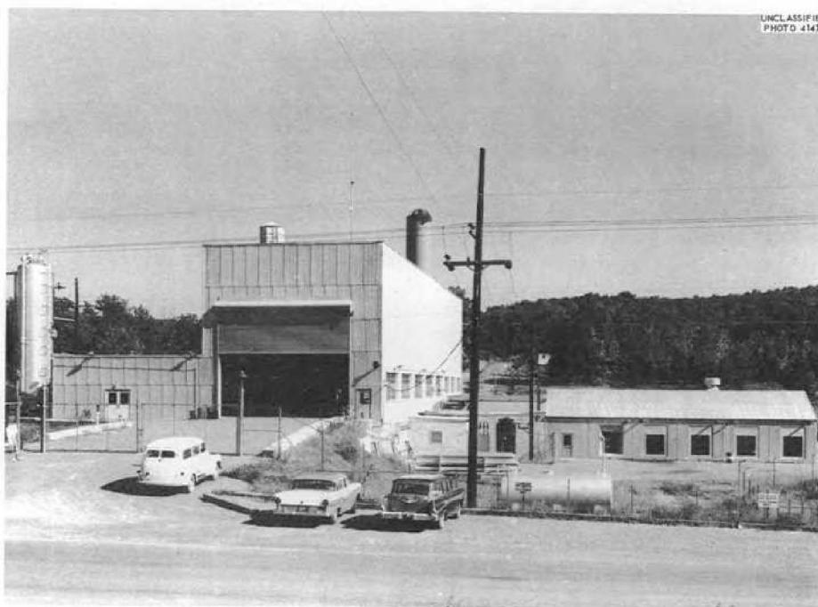
Fig. 21. View of the ART Facility from the Northwest. Photograph showing the status of the facility in August 1957. In the right foreground can be seen the diesel oil storage tank. On the right of the main building can be seen the nitrogen storage facility, the 1500-kva substation, and the diesel generator building. On the left can be seen the process water tank. The 750-kva substation, which cannot be seen in this picture, is directly behind the water tank.
