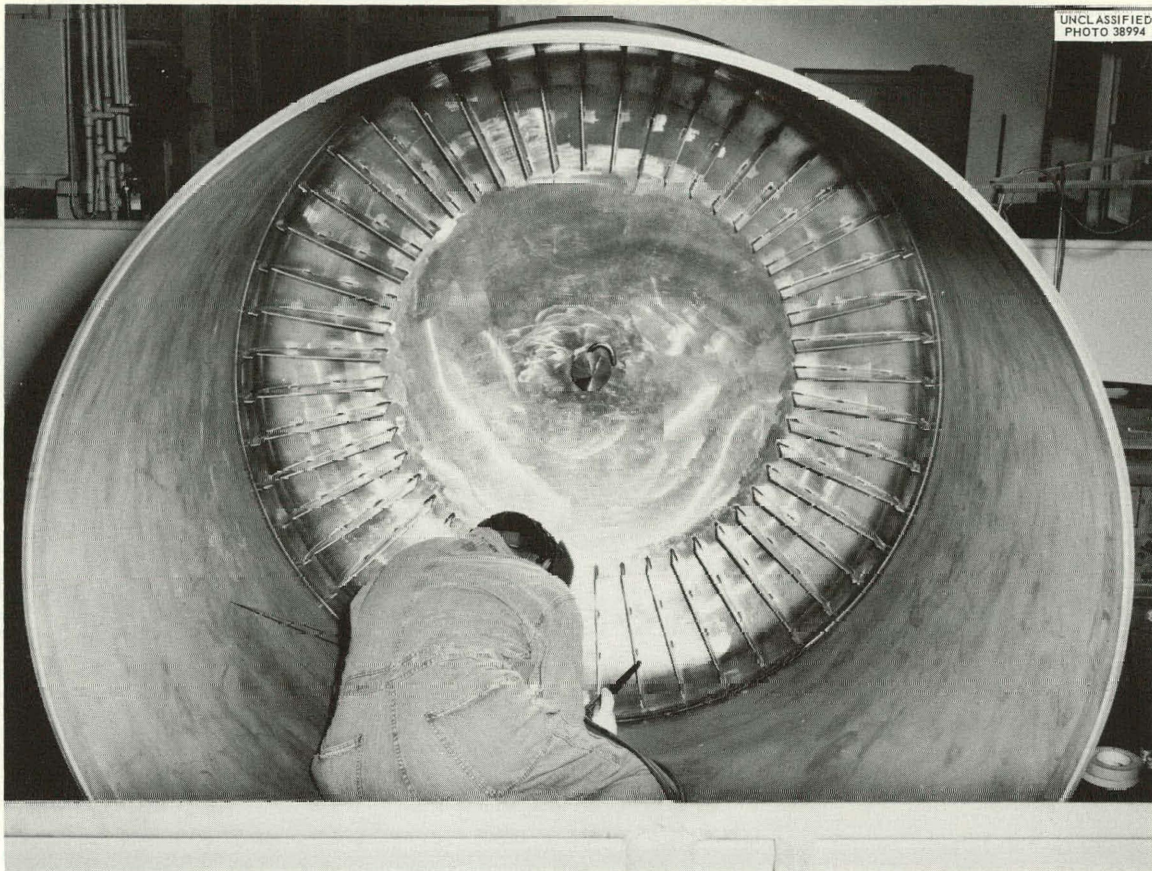
Fig. 1.3. Inside of Reactor Vessel Showing Flow Straightening Vanes.
