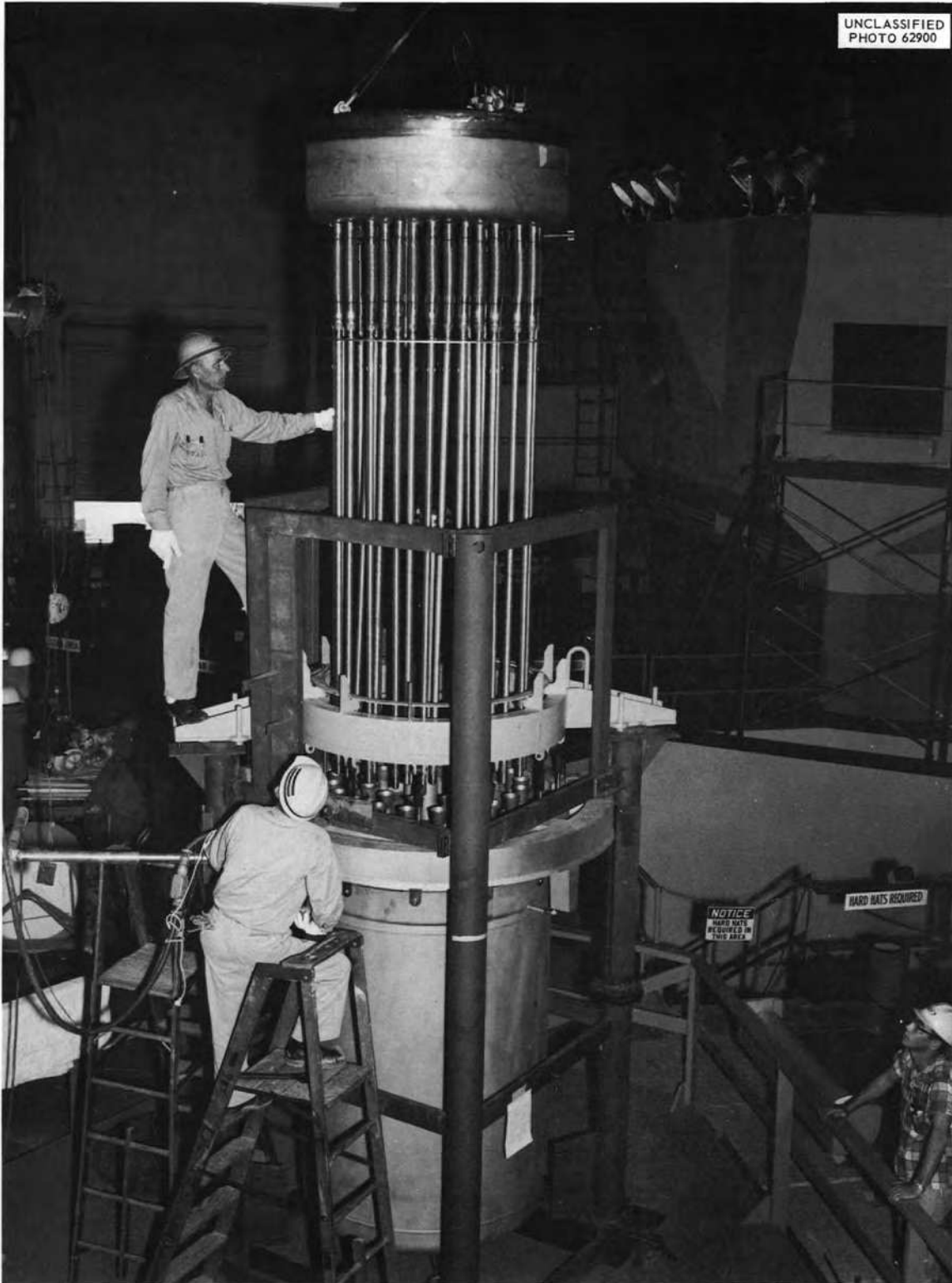
Fig. 1.7. Fuel Drain Tank and Cooler Being Assembled on Jig.
