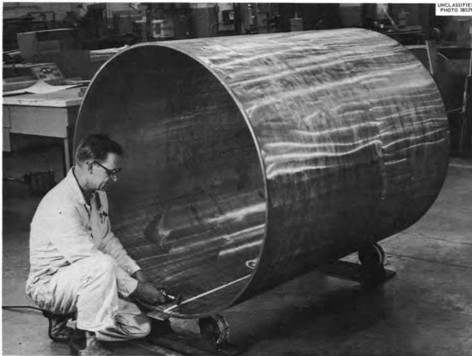
Fig. 22. Typical Rolled Shell for Fuel Drain Tank.
