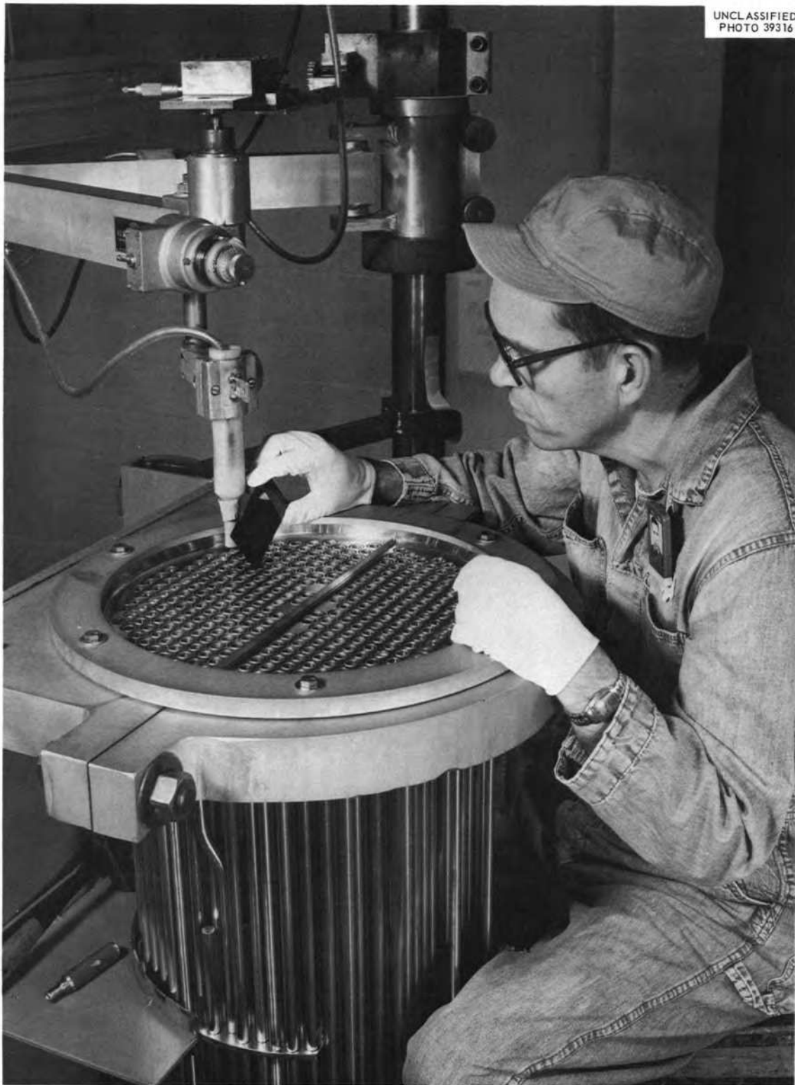
Fig. 28. Welding Heat Exchanger Tubes to Tube Sheet.
