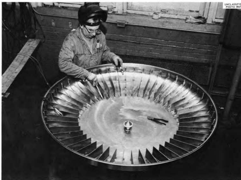
Fig. 37. Attachment of Flow-Straightening Vanes to Reactor Vessel.
