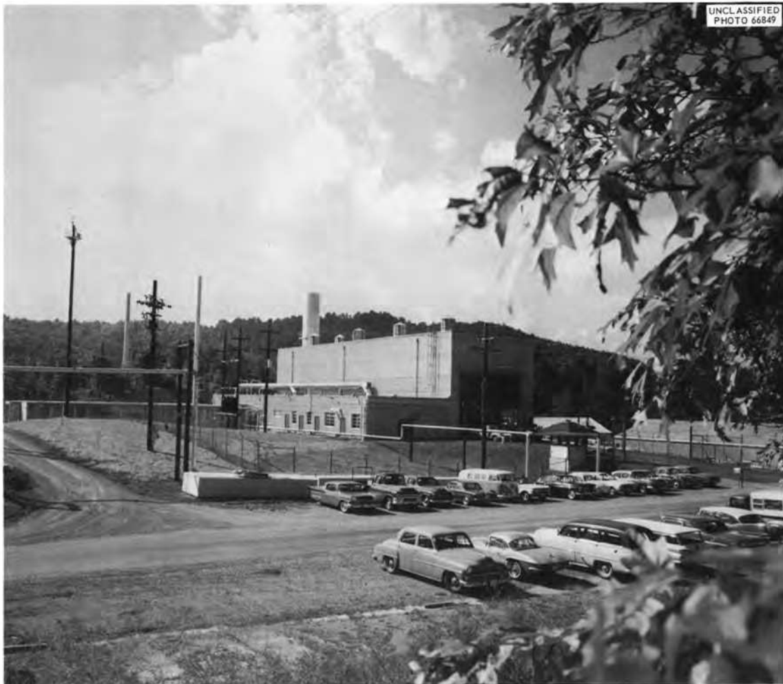
Fig. 7. North View of Building 7503.
