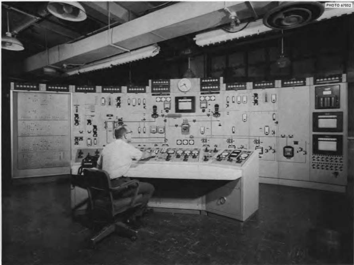
Fig. 1.3. MSRE Main Control Room Panels and Console.
