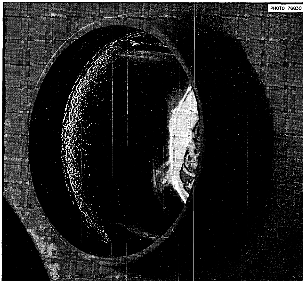
Fig. 3.2. Photograph of Test Freeze Flange Showing Fluorescent Dye-Penetrant Indication of a Crack on the Left Side of Bore.
