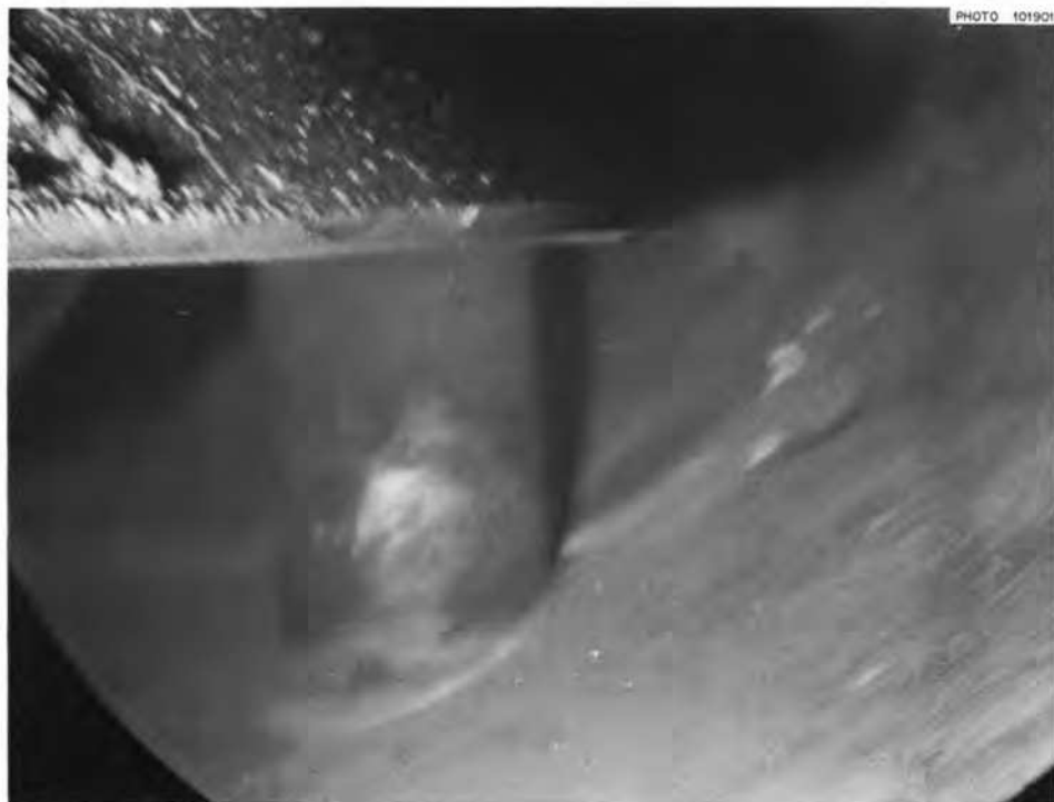
Fig. 1.9. View inside fuel pump bowl showing edge of spray baffle, with scattered deposits. The overflow pipe is visible in the background.
