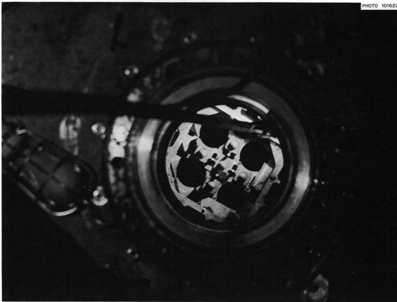
Fig. 1.3. View of top of core through access opening.
