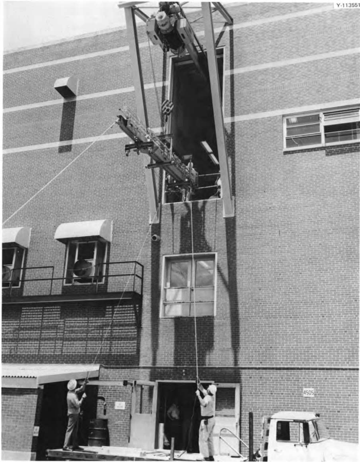
Fig. 34. Mockup and assembly jig being lifted into the room above the experiment cell.
