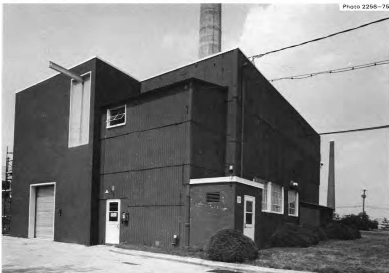
Fig. 6.1. Molten-Salt Test Facility (Building 2011) from the west side. The newly constructed air lock is on the left.
