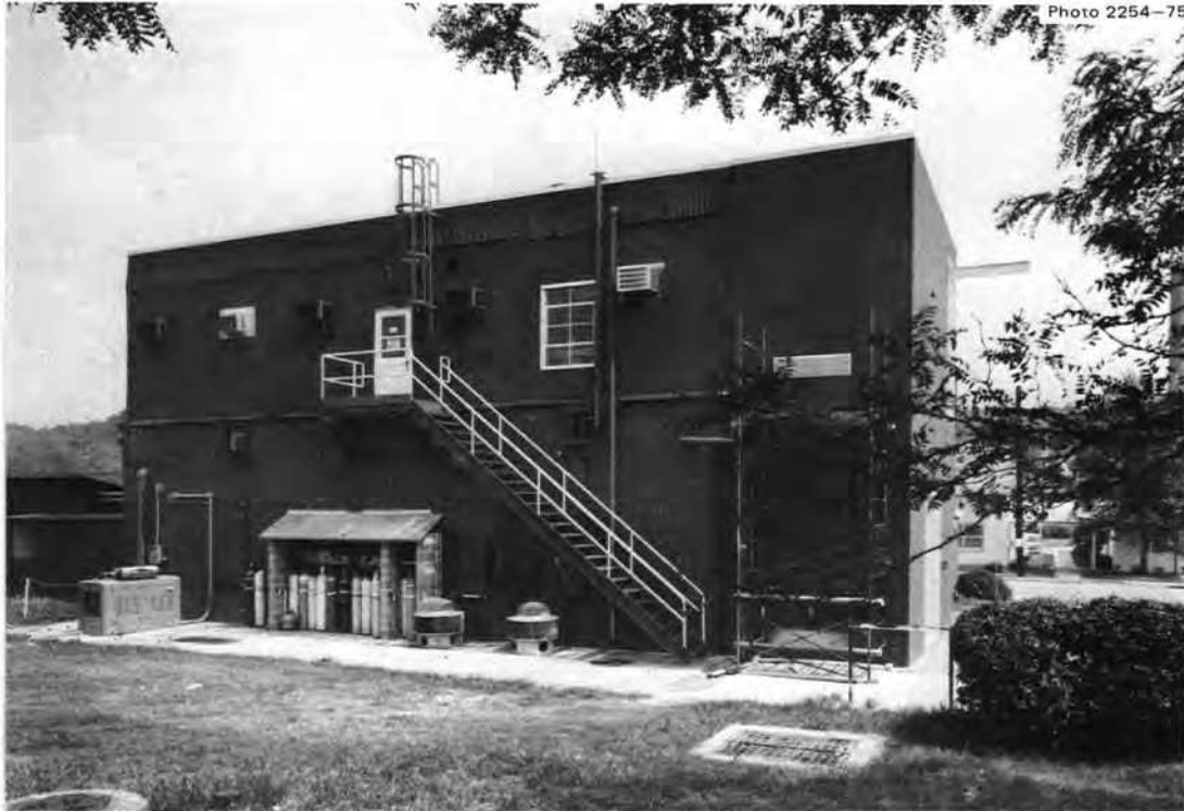
Fig. 6.2. Molten-Salt Test Facility (Building 2011) from the north side. Features of interest include the shop area on the extreme left, the emergency generator on the left, gas storage rack in the center, and the newly constructed air lock on the right.
