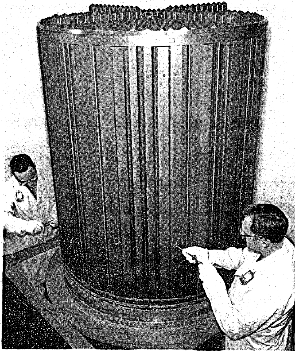
Fig. 25. Anisotropic, Needle-Coke Graphite Grade CGB Being Assembled for MSRE Core.
