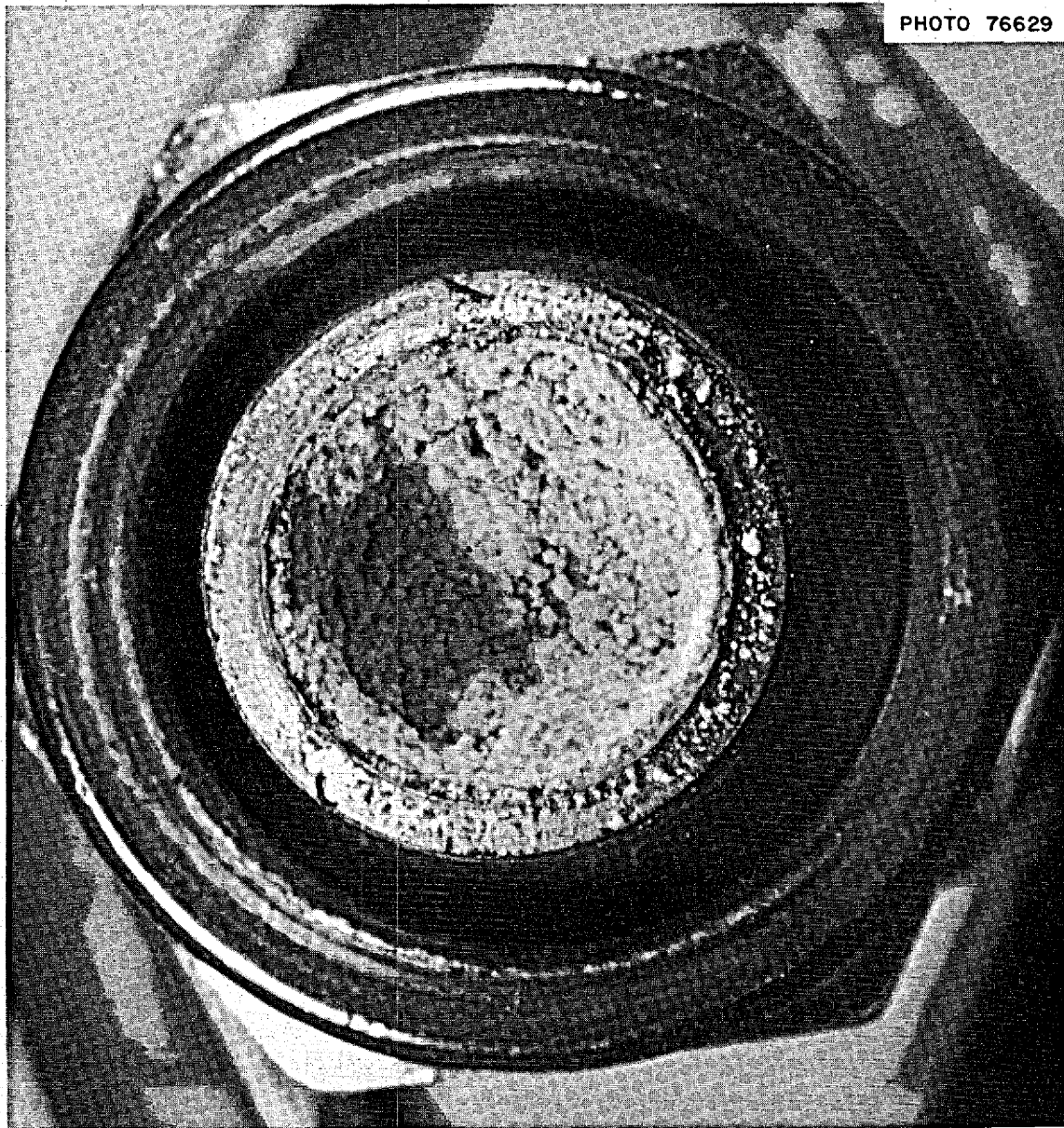
Fig. 28. Salt plug found in 5 1/16-in. line at filter inlet, Mar. 7, 1969. \text{NaBF}_4 circulation test, PKP loop.
